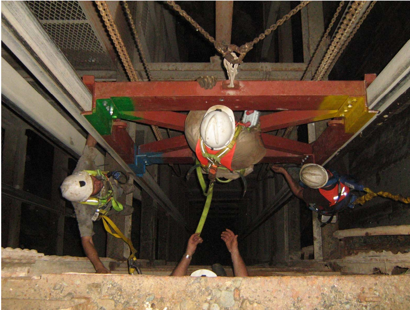
FITTING OF ROPE CENTRING CROSSHEAD
