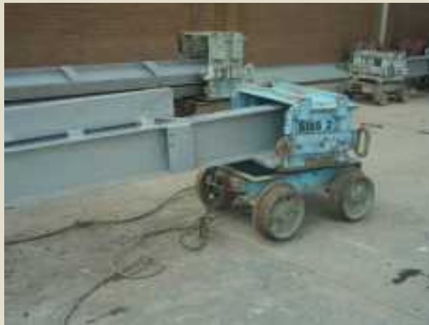
Transport sling too long
