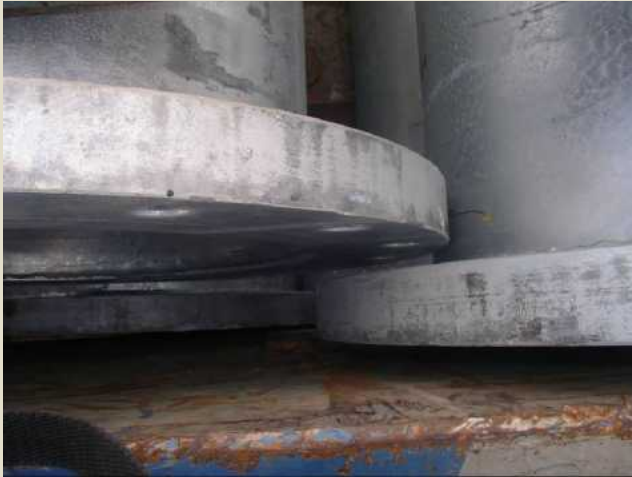
Pipes loaded to ensure symmetry
